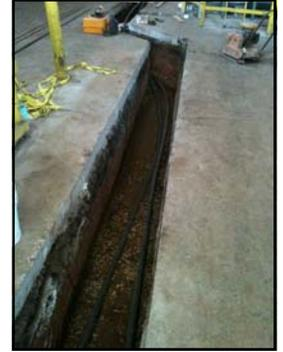
A trench was dug to install better drain lines from the vacuum area and 389-399 tanks to the tower and waste water pits and also to install cooling lines from 952 chiller to 389-399 tanks.
